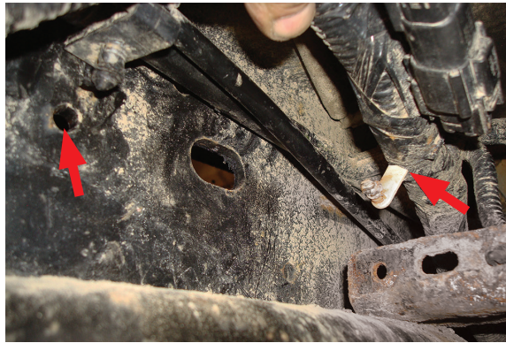
Image shows lines clear on the frame opening it up for the brace installation.
