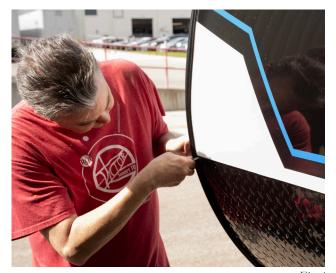
5. Route the Indicator Light's wire through the drilled hole (Fig. 5).
